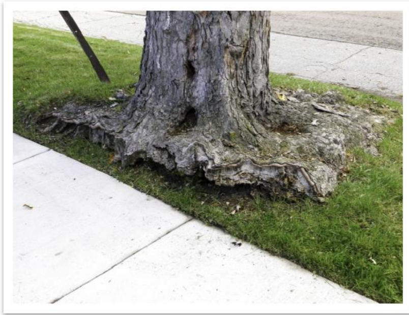
Photo 4 A silver maple noted with both Mechanical Damage and Root Problem due to excessive root pruning during sidewalk reconstruction.
